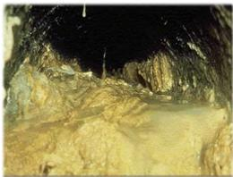
Grease buildup on the interior of sewer line.
